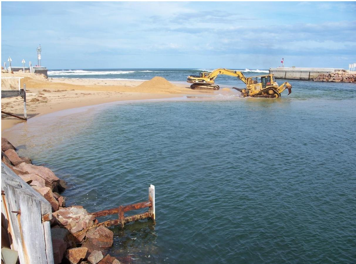
*Figure 3: Entrance Channel severe sand accumulation in May 2007 (Lakes Entrance)*
