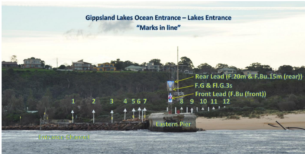
The photo above is taken from seaward of the Entrance and illustrates the “Leads in Line” when the “front Lead” is located on the “Green Light”
