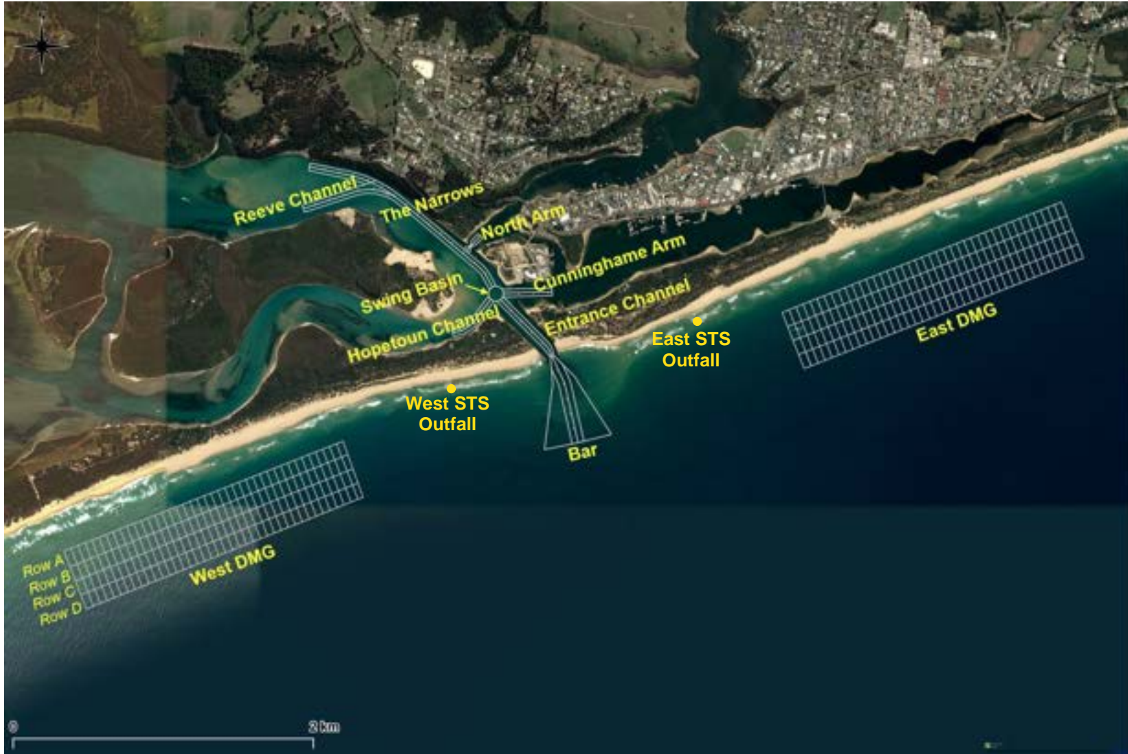
Figure 1. Port of Gippsland Lakes dredged areas and DMGs.
