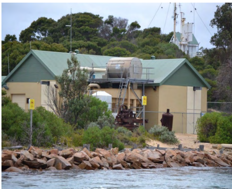
Figure 52: Sand Transfer Station pump building
